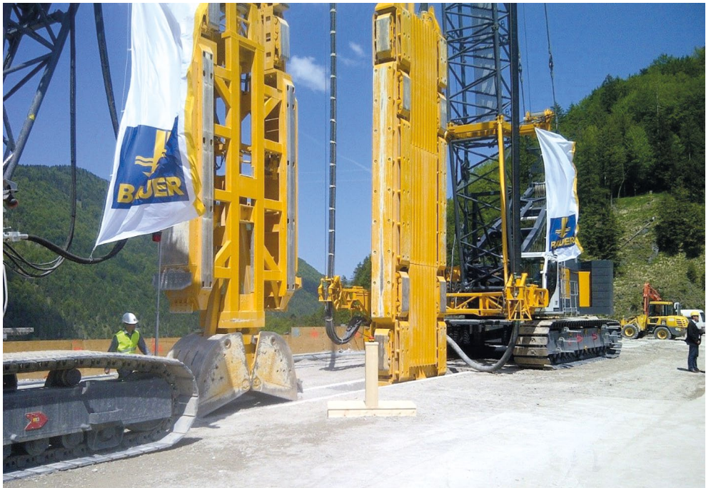
Fig. 1. Main equipment for the cut-off wall installation – BAUER DHG Hydraulic Grab (left) and BAUER BC40 Trenchcutter (right).
