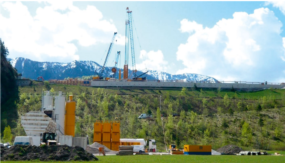
Fig. 3. Concrete batch plant at the downstream side of the Sylvenstein dam.
