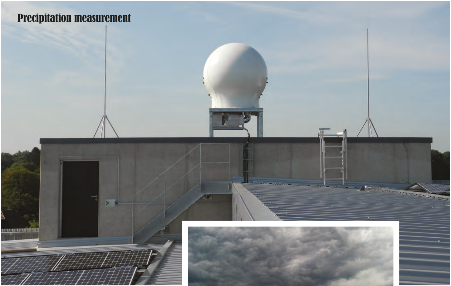
ABOVE: A GAMIC X-band weather radar installed on top of a parking structure south of Aachen, Germany
