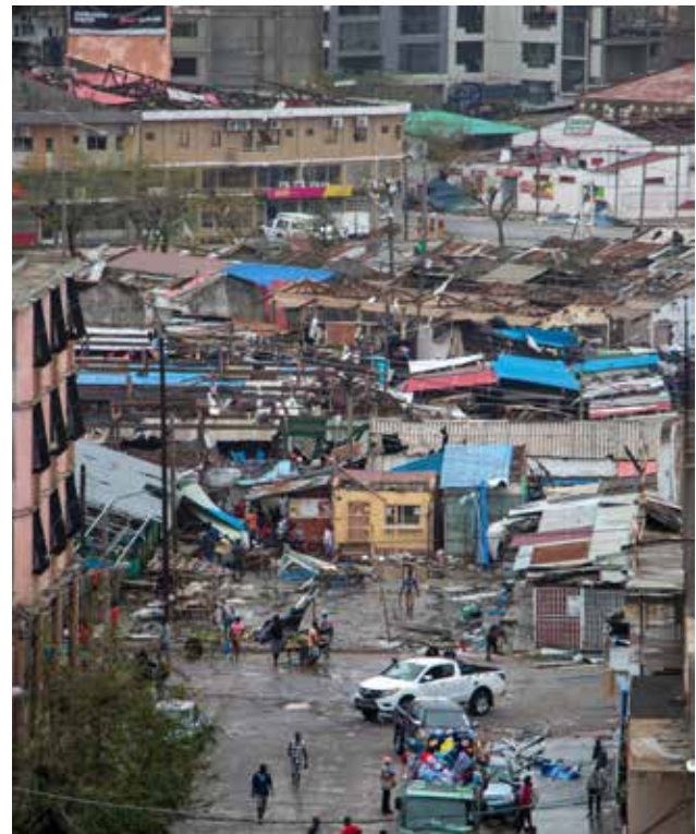
Figure 4. After the passage of the strong Cyclone Idai, the trail of destruction left in Beira City was very visible. The roofs were simply pulled out, nothing was the same! (Source: iStock/ Duarte Gouveia)
